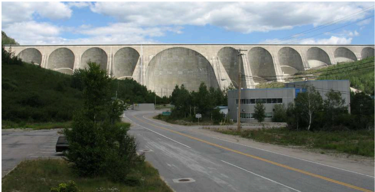
Daniel-Johnson Dam in Quebec, Canada with buttresses
